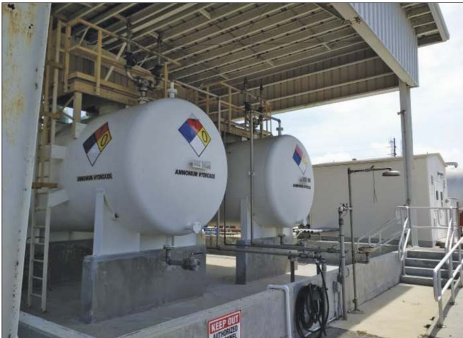
Figure 1. Bulk Tanks and Metering Pump Building
