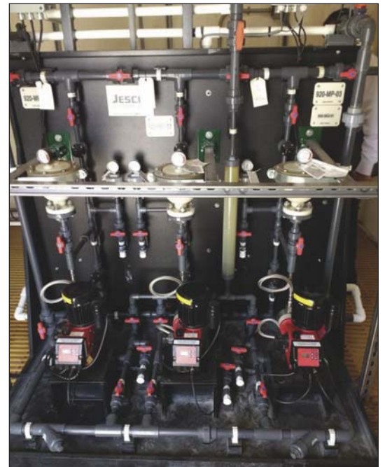
Figure 2. Metering Pump Skid
